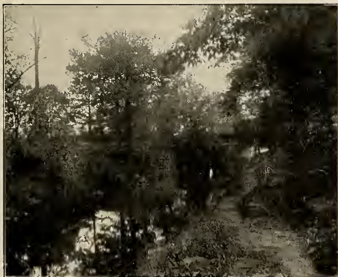
The crumbling piers of the Old Bergen Road Bridge
